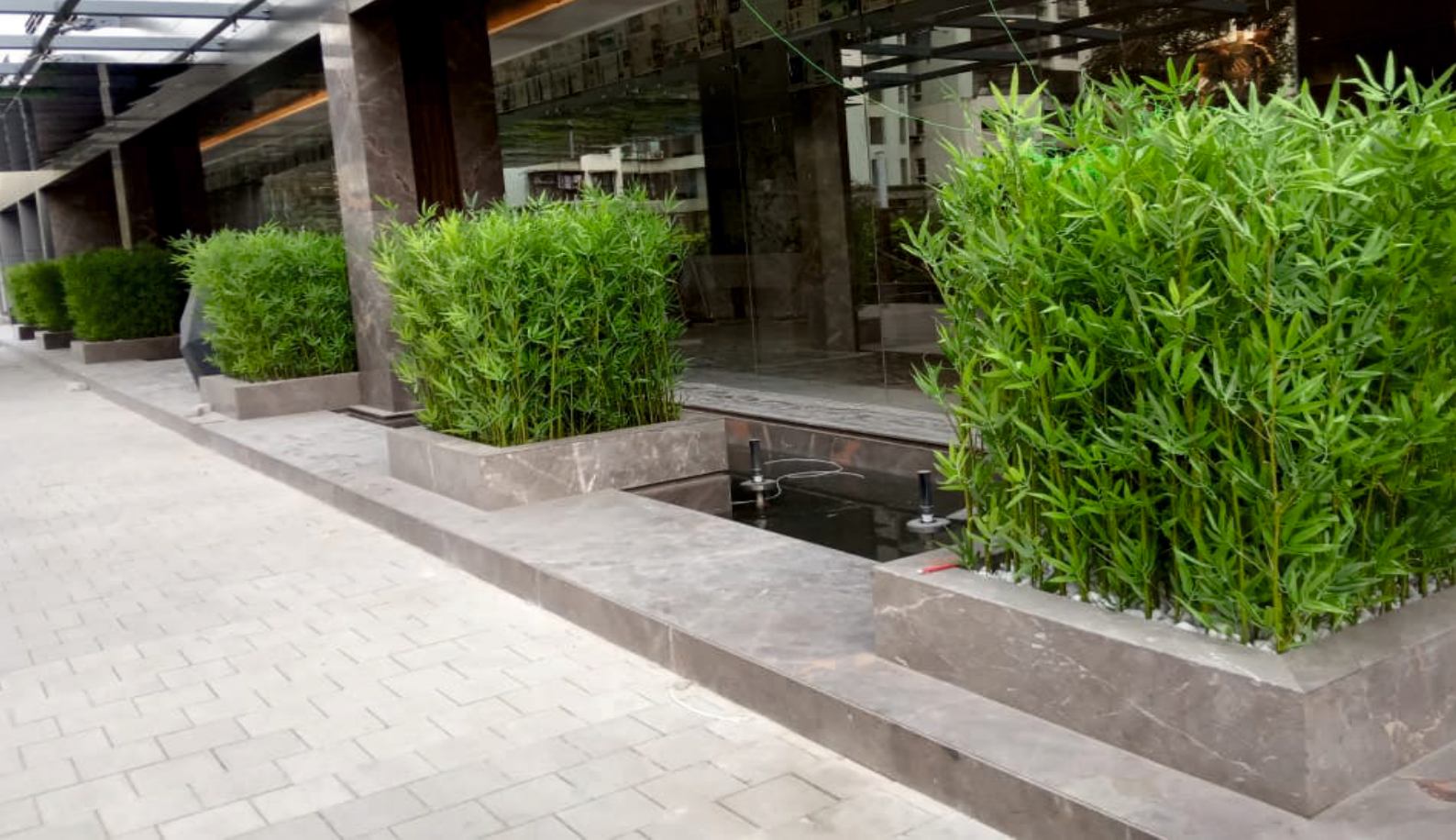
At this site we used 420 Bamboos of 8.5 feet height (3742 B), cut them into 2 and installed 140 Bamboos per pocket. Thereafter we covered them with polished marble stones. The Real Touch leaf added beauty to the entire installation done outdoors.
